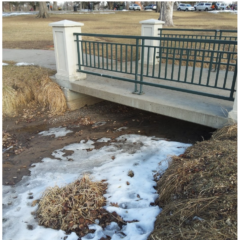
Photo of the bridge and ditch in current state
