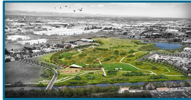
Late 2023 | Heron Pond/Heller Open Space Regional Park Ecosystem construction complete (7.37 Habitat Units of 87.4)
