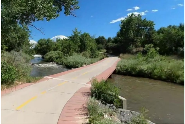
Photo shows example low flow bridge structure.
