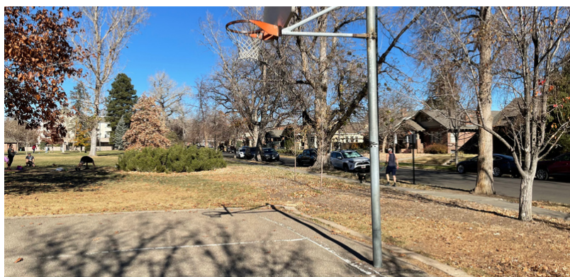
Existing Basketball Court To Be Replaced
