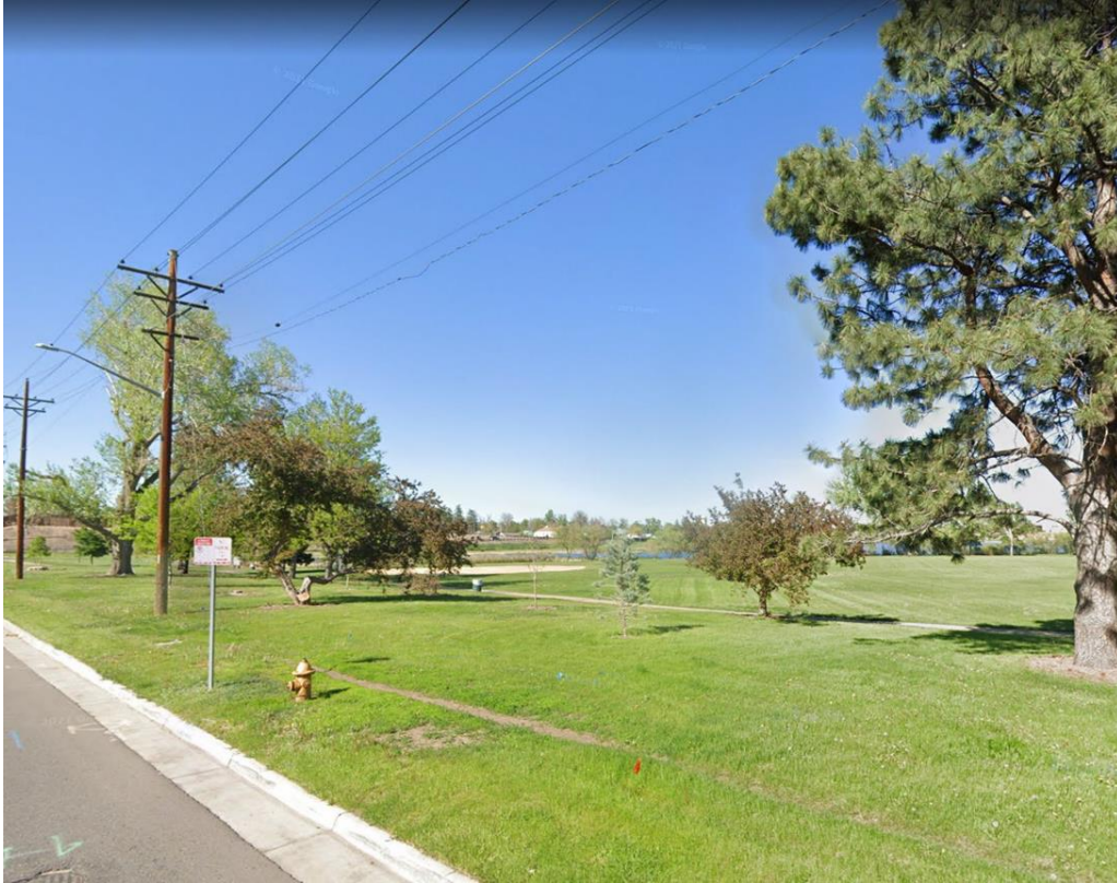
2.1.1.b - Low traffic areas along the right of way that have utility lines buried and are not suitable for tree plantings.
