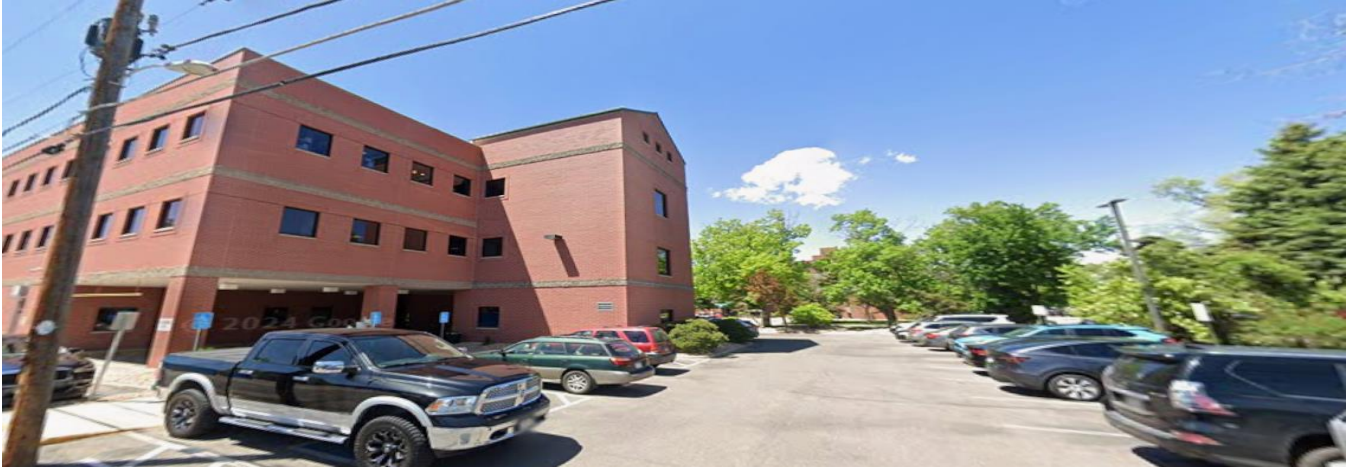
View from alley between East 18 th and 19 th Avenues, looking north (via Google Earth)
