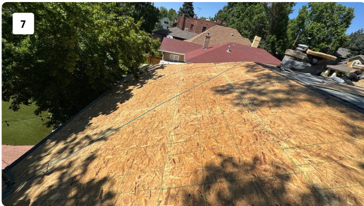
New decking installed on all slopes
