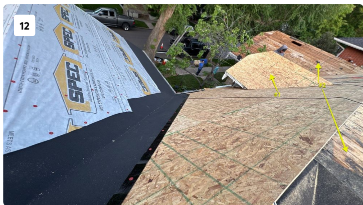
#1 New decking #2 Old decking
