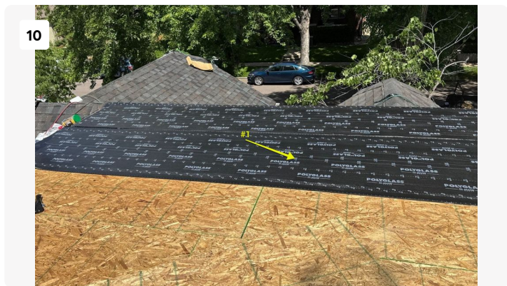
#1 - New base sheet installed under new top sheet
