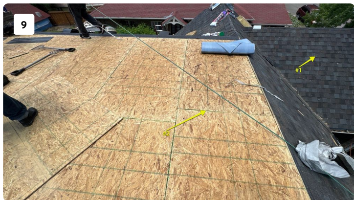
#1 - New Black walnut shingles #2 - New decking
