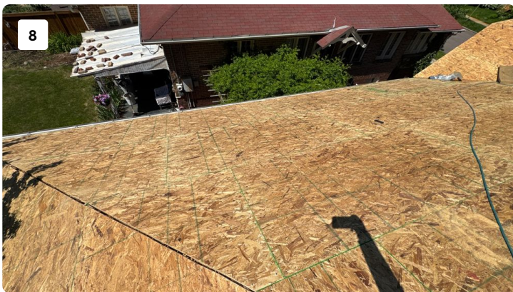
New decking installed on all slopes
