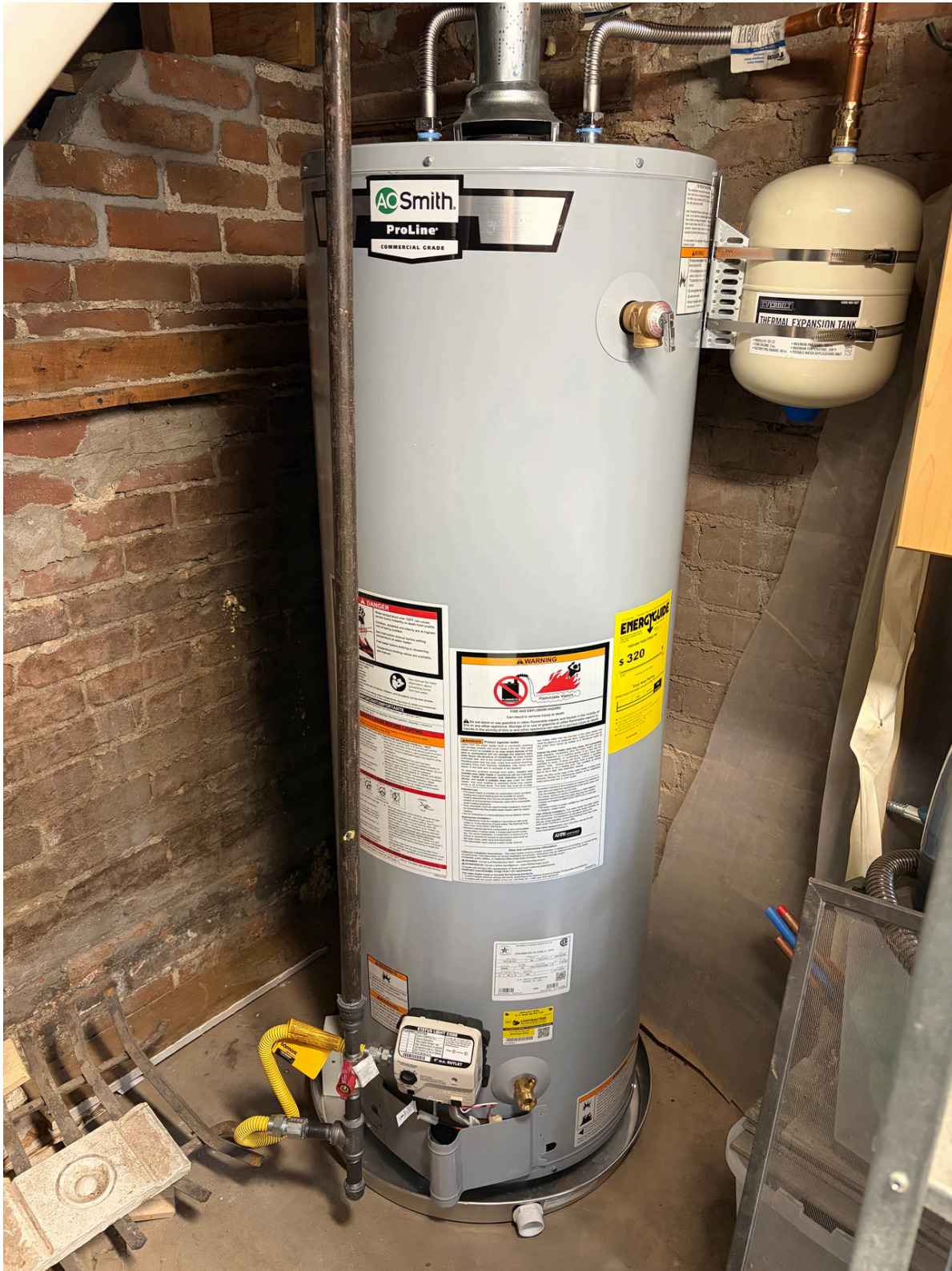
Completed Water Heater Install (photo 3)
