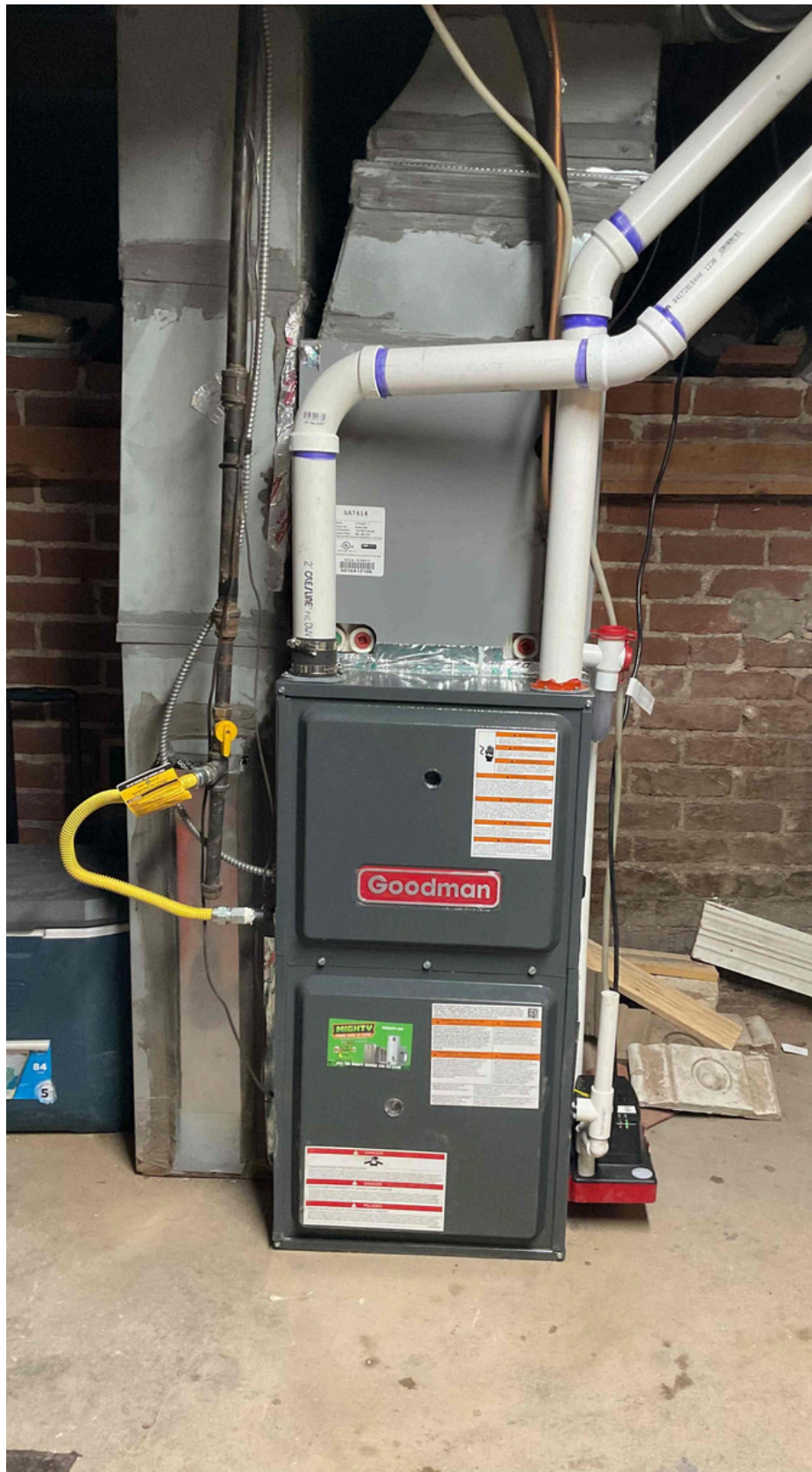
Completed Furnace Install (photo 2)
