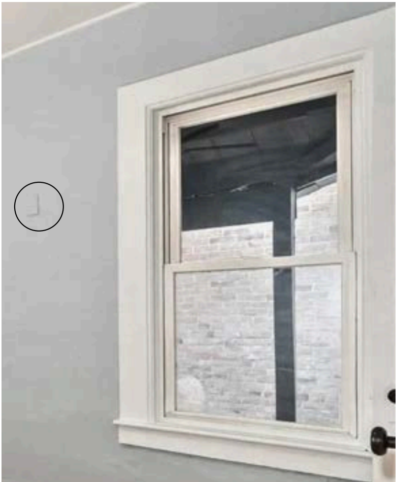
51. Switchplate cover and unoriginal window trim on South facing window
