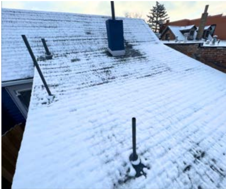
30. Wide view of chimney/roof
