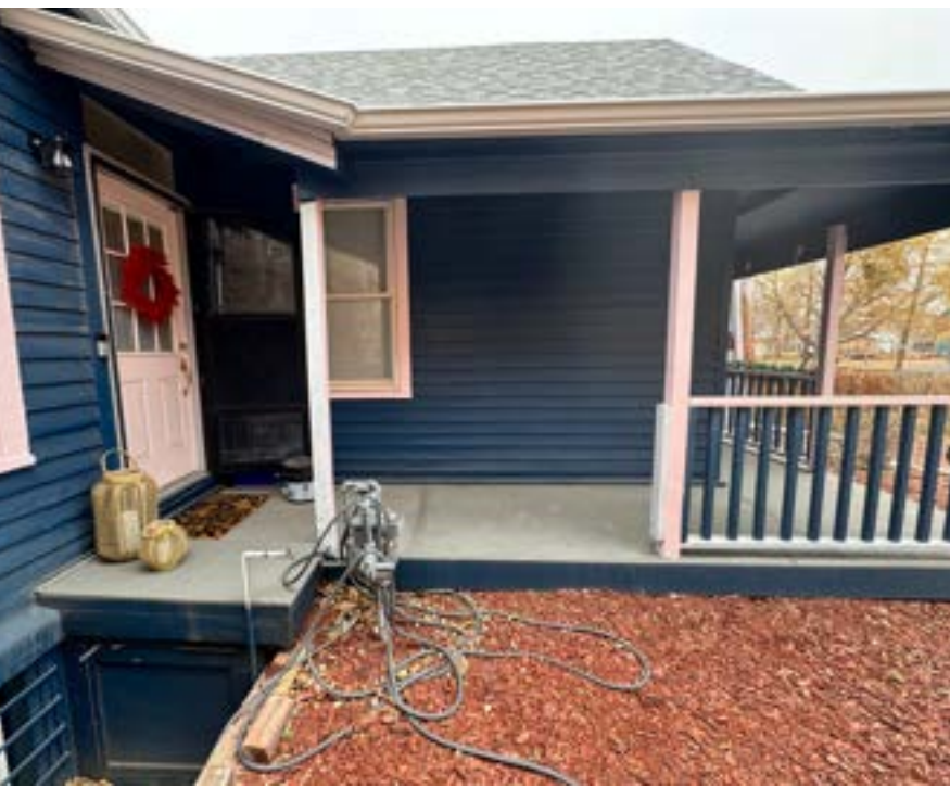
3. Left view of porch (facing North)
