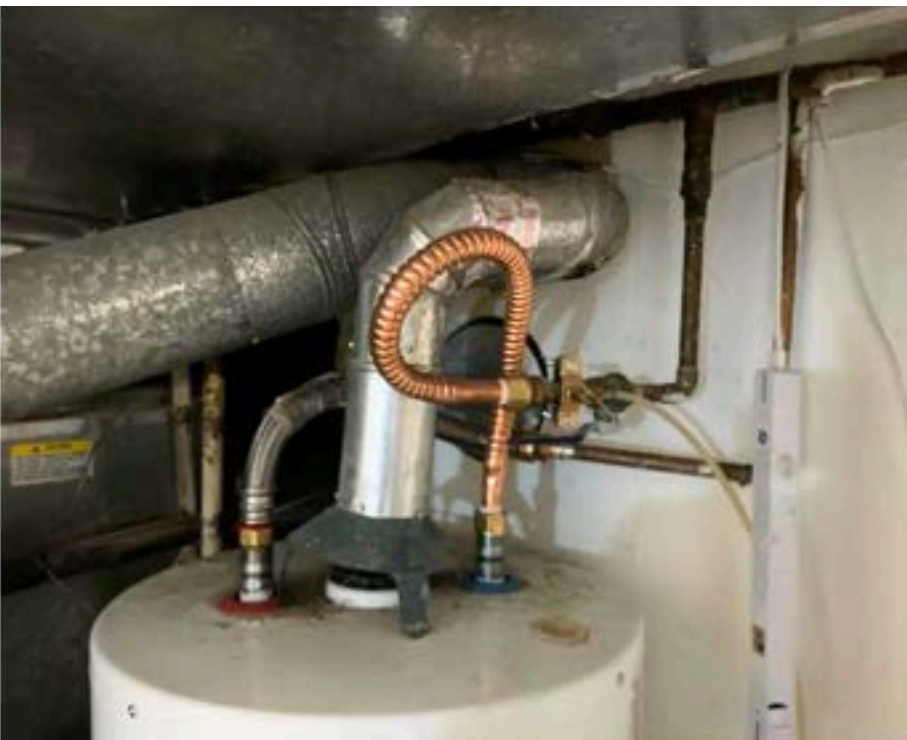
33. Flue venting connections
