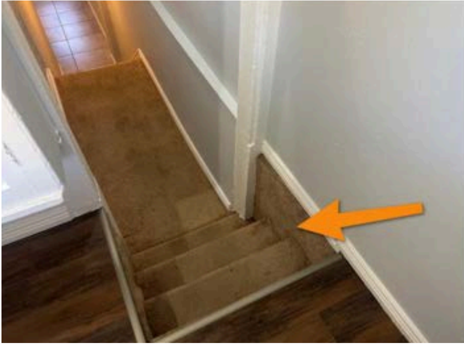
60. Basement stairway (note carpet) East view
