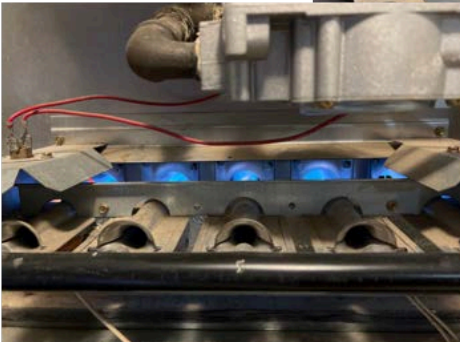
26. 5 Burner detail of furnace
