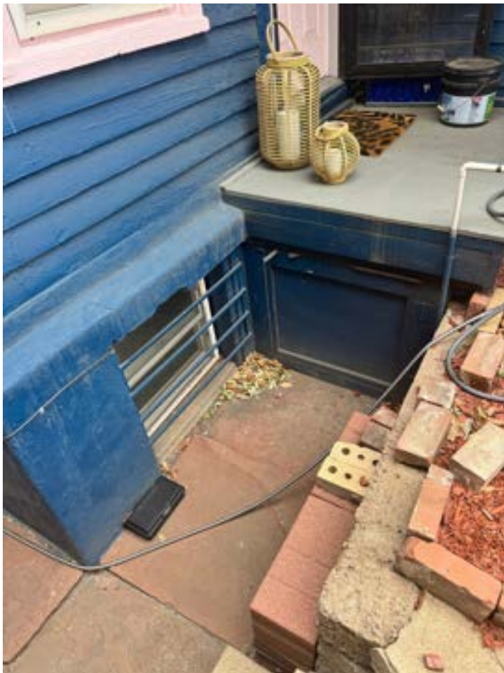
5. Left side of house (Facing west), basement egress window
