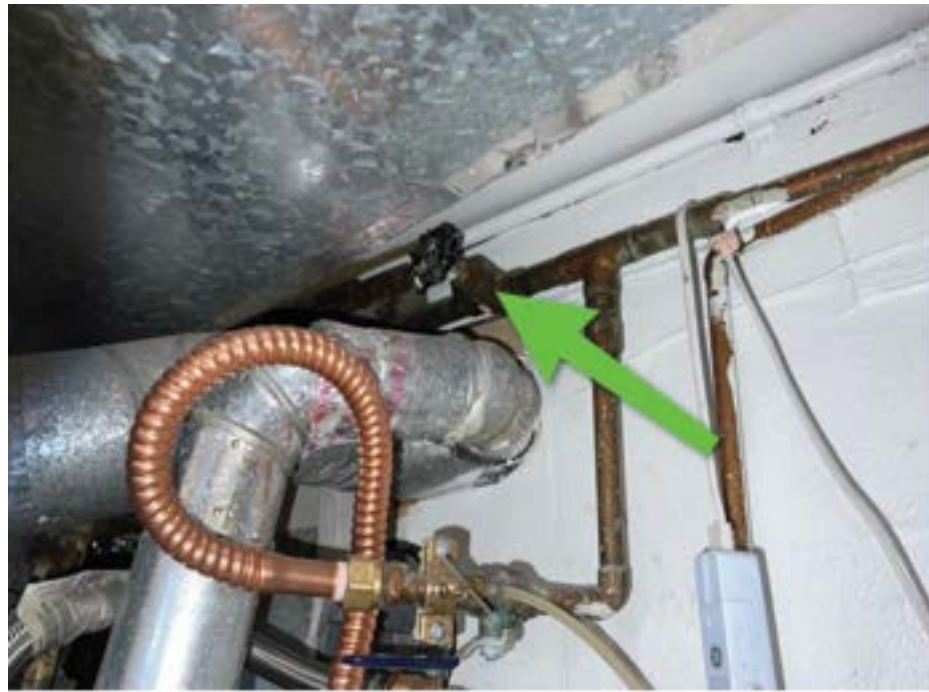
32. Main water shut off
