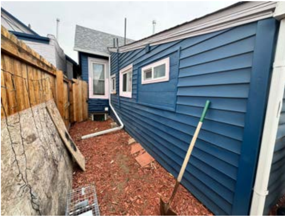
11. Right side of house (facing East)
