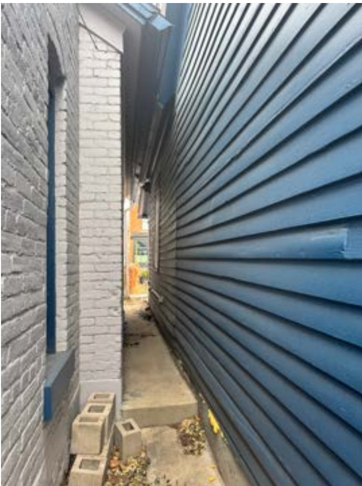
8. Right side of house (Facing East)
