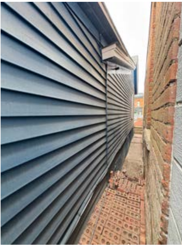
6. Left side of house (facing East)
