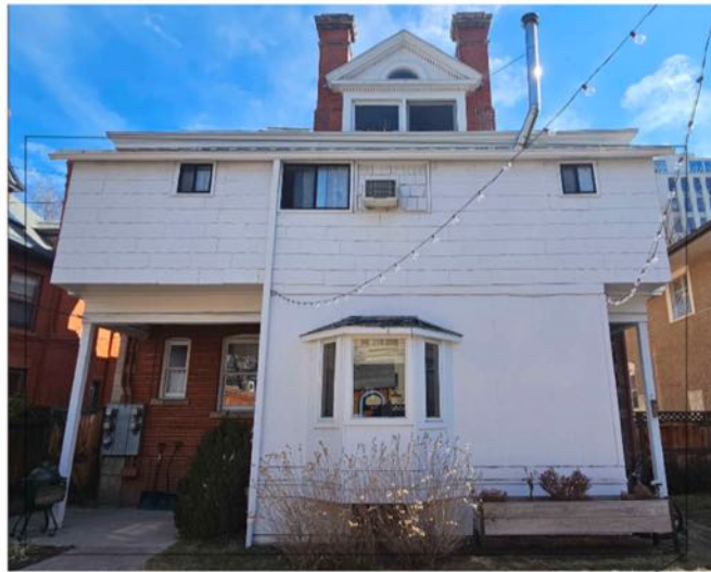
EXISTING WEST ELEVATION VIEW FROM WEST FROM REAR YARD
