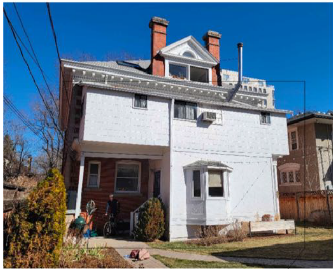
EXISTING NORTHWEST ELEVATION VIEW FROM NORTHWEST CORNER OF REAR YARD
