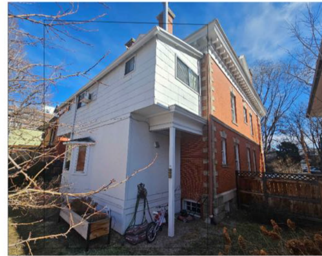
EXISTING SOUTHWEST ELEVATION VIEW FROM SOUTHWEST OF REAR YARD
