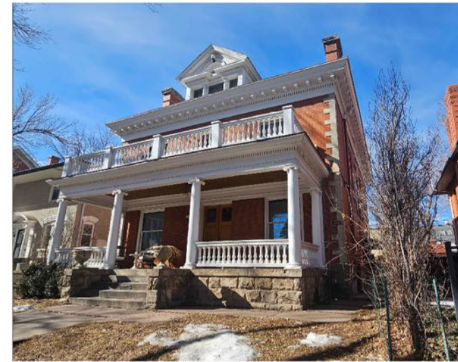
EXISTING NORTHEAST ELEVATION VIEW FROM NORTHEAST CORNER ON HIGH STREET
