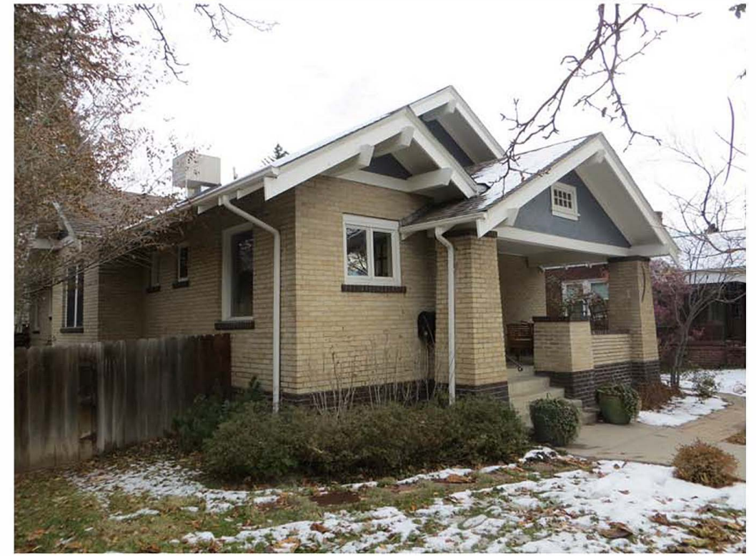
HOUSE FROM NORTHWEST
