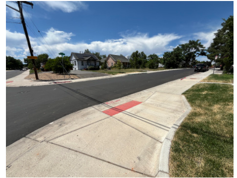
Wide sidewalks replace gravel shoulders and improved drainage was installed.
