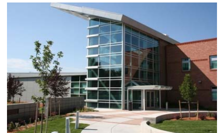
District 3 Denver Police Station
