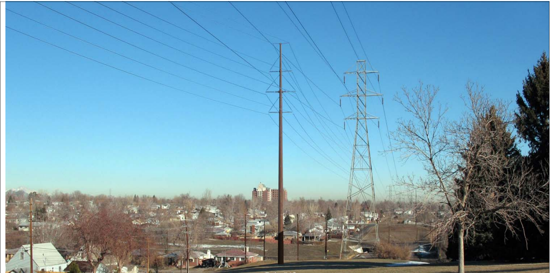
Electrical power lines cross Ruby Hill Park, as they do in many Denver neighborhoods. Xcel Energy wants to replace the older lattice towers, as seen on the right, with newer single poles like the one on the left. The new line would have less visual impact but would violate the view plane ordinance. Building the line above-ground would cost $600,000. Burying it, as Ruby Hill residents want, would cost $5 million.
