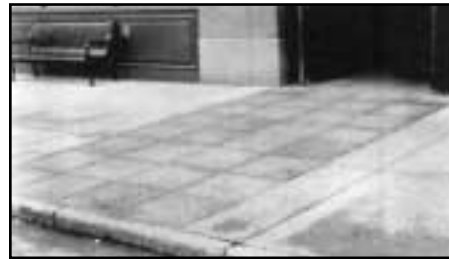
Flagstone paving "welcome mat" at the entrance to the Oxford Hotel. MacIenman 1991
