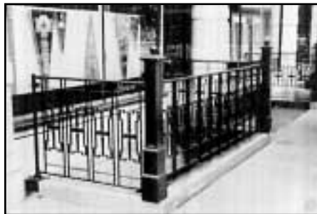
Railing at the Oxford Hotel annex.
