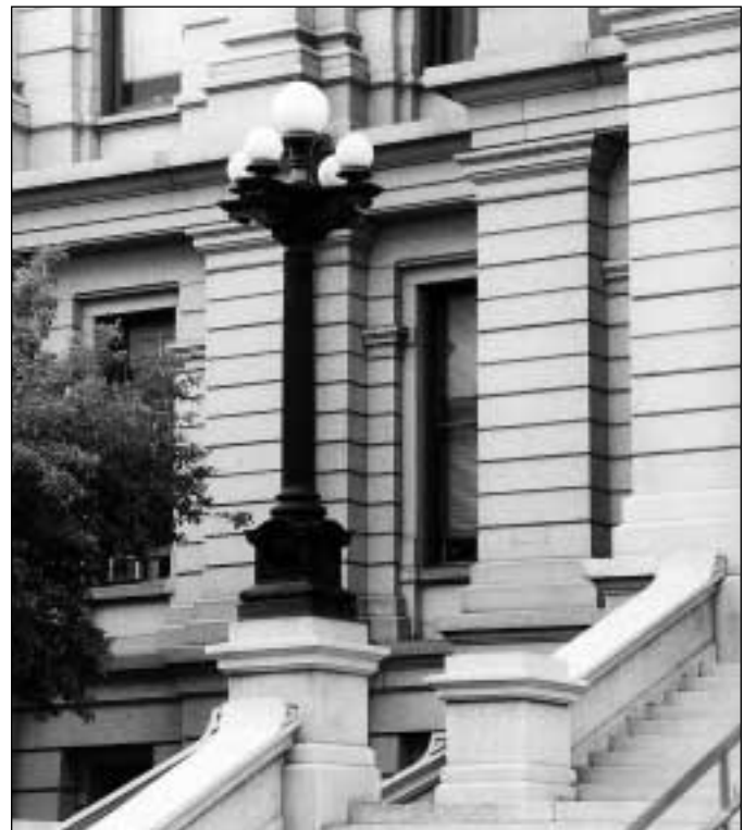
Stairs to heroic buildings deserve heroic newel fixtures. This qualifies.
