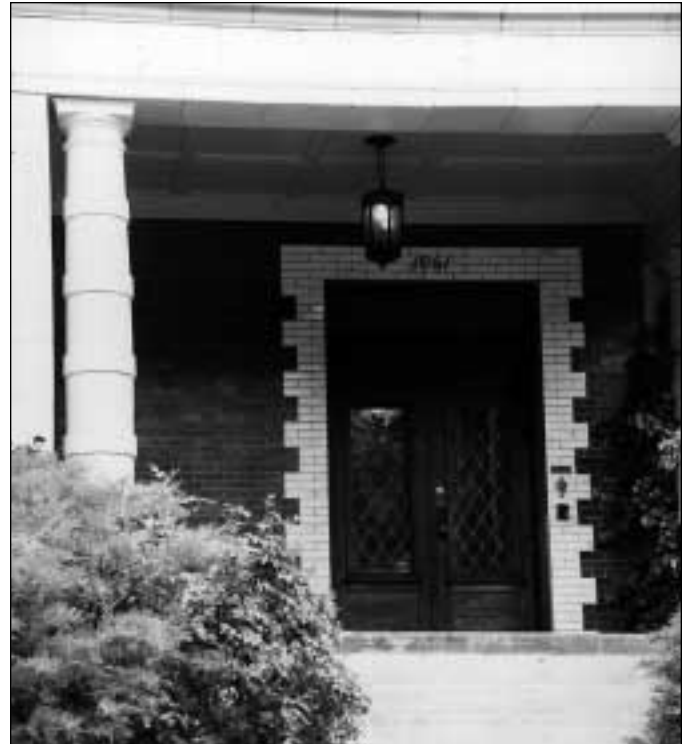
Fixtures at the building entry are the first call for night lighting. Porch ceiling-surface or pendant fixtures are typical for historic residences once owned by either rich or poor.
