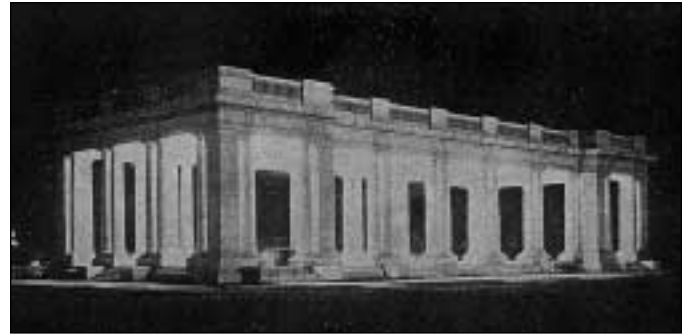
The Cheesman Memorial gleams from within from largely concealed sources. The building is a lantern for the park. Courtesy Denver Public Library, Western History Department.
