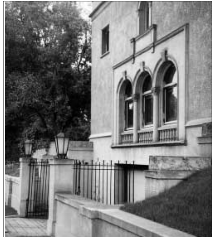
Individual property lights at the fence lines enhance the night character of residential districts.
