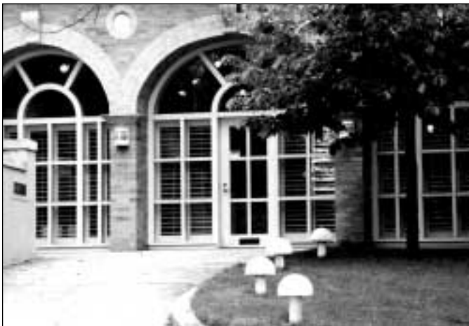
The arch-pier sconce lights and the path lights are clearly additions in this rehabilitation but in sympathy with the historic structure. They are appropriate in the adaptive use of this site.
