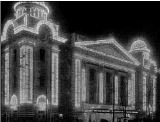
The Denver Auditorium defined the structural organization of the building with light at night. Courtesy Denver Public Library, Western History Department.
