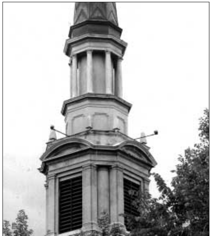
The steeple of this church is a significant Denver landmark, and is properly lit with floodlights on outrigger arms as well as with lower roof-mounted sources.
