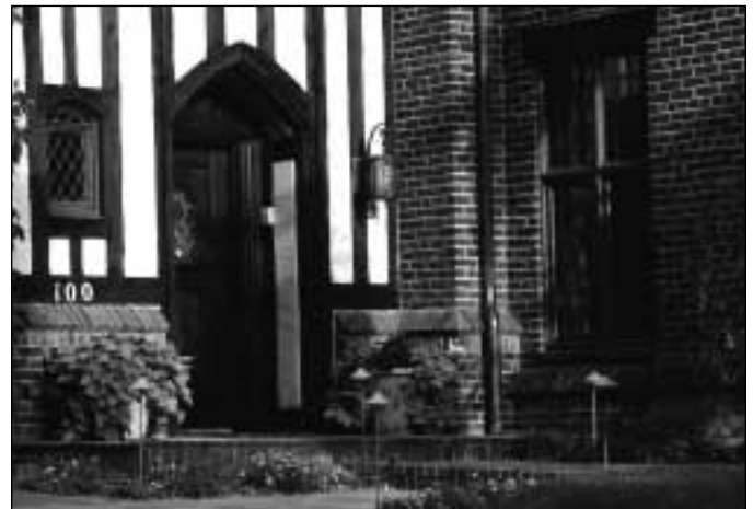
The five path lights are low-keyed means of lighting the pathway steps without upstaging the historic entry lantern.
