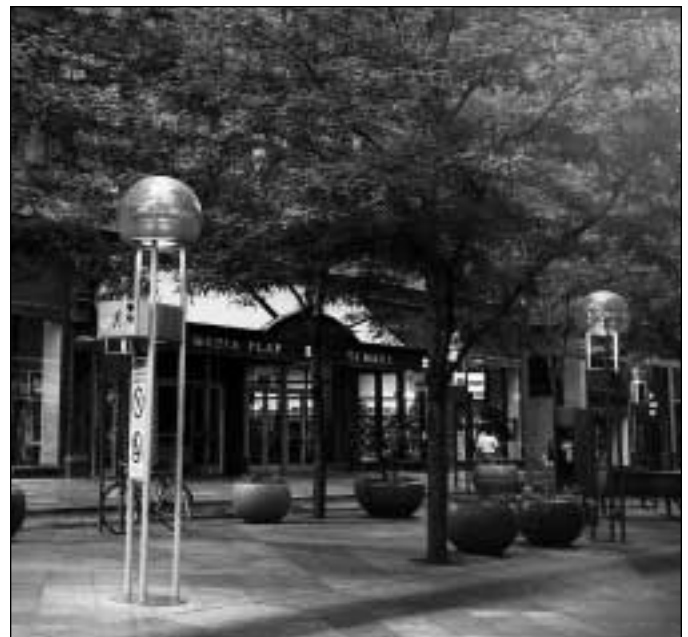
The 16th Street Mall lights are an outstanding design and effectively provide general illumination without glare, with sparkle that simulates with fiber-optics the output of incandescent lamps. The sources are metal halide HID lamps that provide good color rendition and economy.
