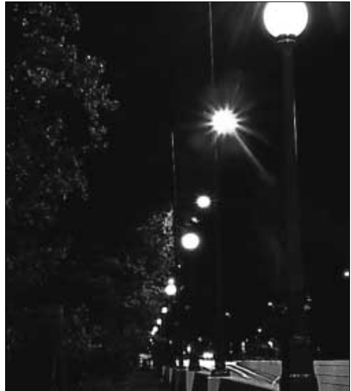
Speer Boulevard. High street lights are lamped with sodium vapor HID's, the lower lights with fluorescents. Photo by Roger Whitacre.
