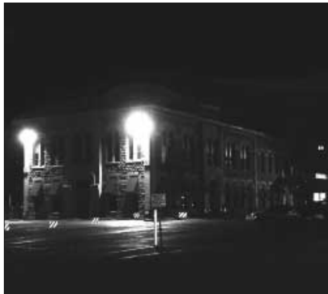
Floodlights placed high for security give rise to the unintended sense of danger and prison-like circumstance. Such lights often create nuisance glare for adjacent properties.
