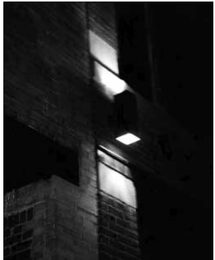
This light at the ground floor cornice line gives useful illumination to the sidewalk below, but adds equal scalloping light against the facade above that is visually disturbing.
