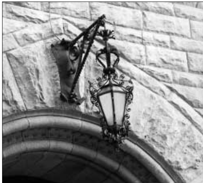
If this landmark entry were not initially provided with this keystone lantern, it would be wise in rehabilitation to seek new illumination from a concealed source.
