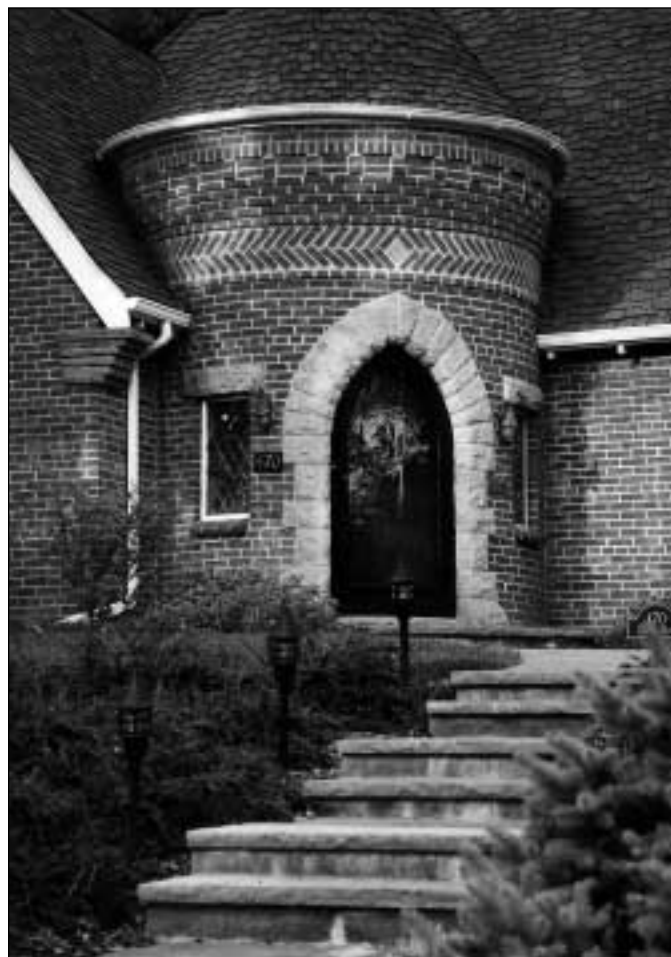
And, in like manner, these stair lights enhance the character of this fine residence.
