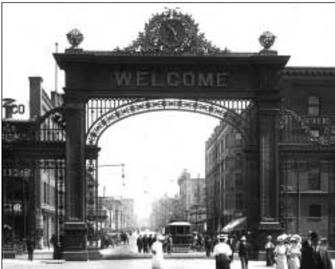
Union Station Welcome Arch, now demolished. View up 17th Street by L. C. McClure. Courtesy Denver Public Library, Western History Department.
