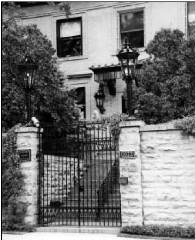
Early electric fixtures evolved in style from gas fixtures. These entry pier and bracket lights could be either gas or electric.
