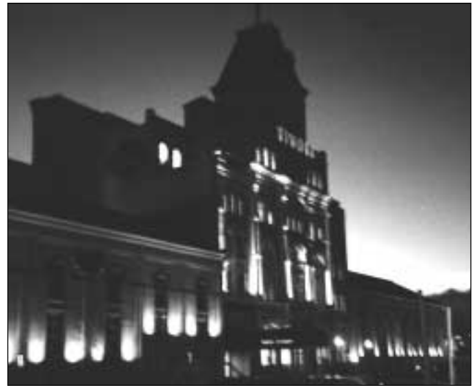
The night time dignity of this landmark industrial building was not well-served in adaptive use rehabilitation for commercial use. Light shining up from above the ground floor is seldom appropriate. Light should shine down at the sidewalk and at entries, not up on the building.
