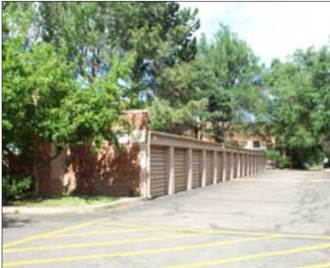
Three garage buildings are located along the south edge of the district.
