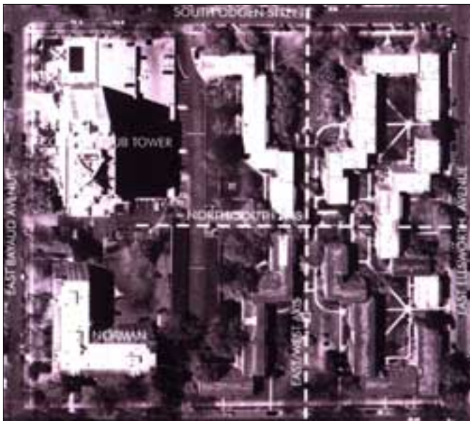
An aerial view of the existing buildings and courtyards.
