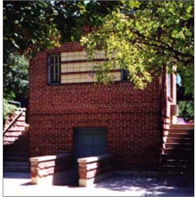
This is an example of an existing secondary structure incorporating some of the same architectural details as are present in the primary structures on the site.
