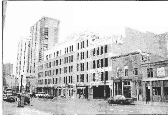
New parking structure in LoDo which reinforces the street edge and the pedestrian friendliness of the area.
