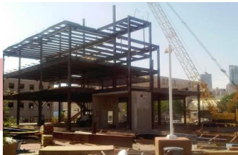
New Police Crime Lab - Construction Progress
