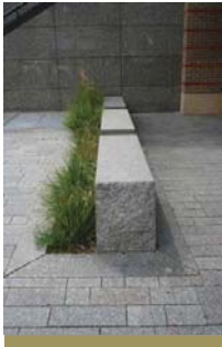
Slab seat walls adjacent to planted beds
