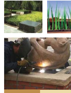
Pedestals for public art can double as seating areas until pieces are installed (a metal welding plate allows for rotation of art elements)
