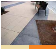
Scored and sand-finished concrete sidewalks are the standard
