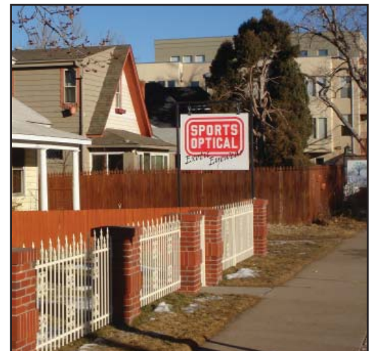
Adaptive reuse of residential properties have resulted in an increase of retail, restaurants and services along Tennyson Street.
