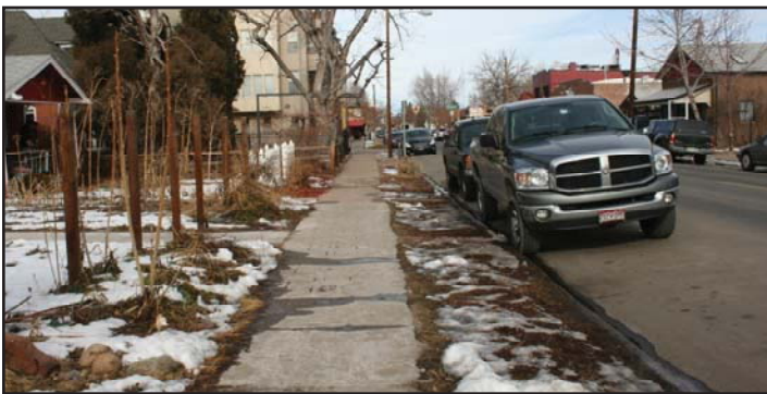
Sidewalk widths between 38th and 44th Avenue vary, but there are several locations where the sidewalk is too narrow to accommodate increasing amounts of pedestrian traffic.
