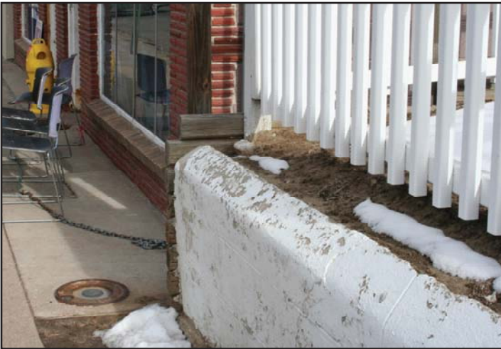
Older retaining walls along the east side of Tennyson Street, across from Caesar Chavez Park.
