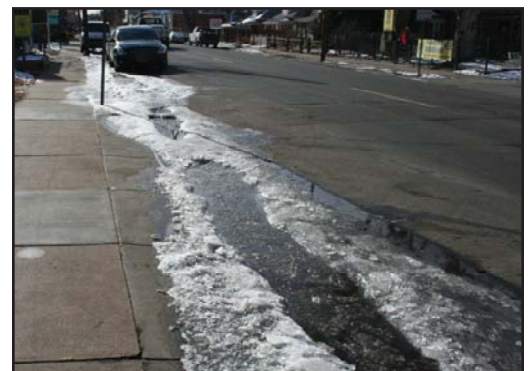
Recent ice damming at the intersection of Tennyson Street and 44th Avenue
