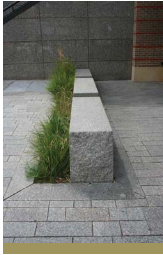
Slab seat walls adjacent to planted beds
