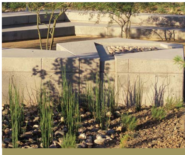
Seatwalls can be used to channel stormwater into adjacent planted beds
