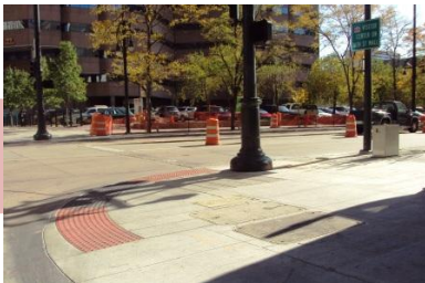
California Street Streetscape and Sidewalk Progress
