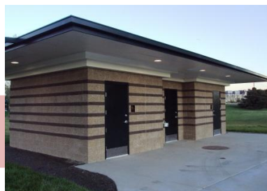
Vanderbilt Park New Restroom
