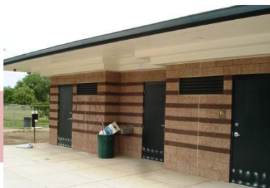
Garland Park New Restroom
