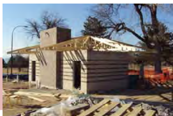
City Park New Restroom - work in Progress
