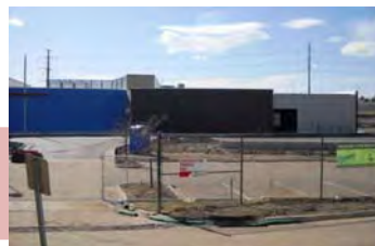
Police Traffic Operations/ Firing Range - work in Progress
