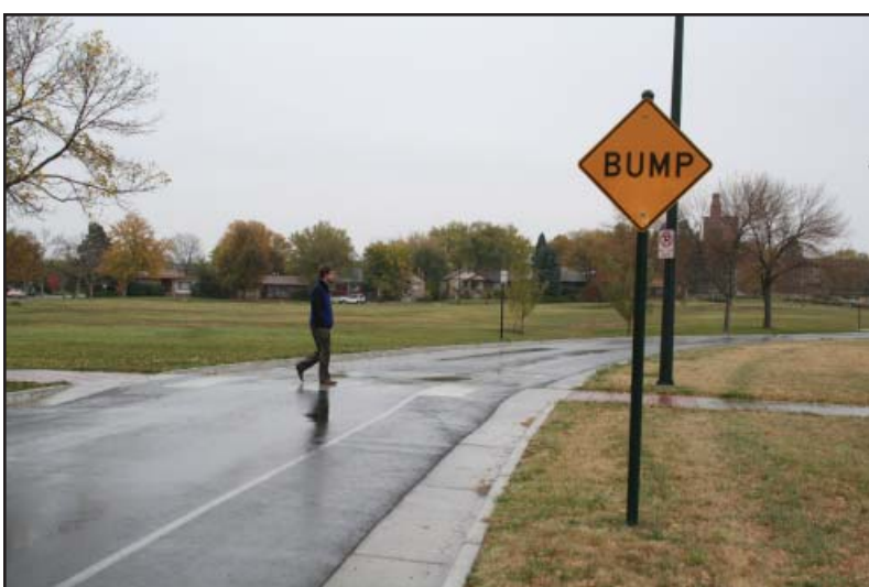
Raised Pedestrian Crossing Table
