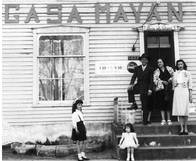
Casa Mayan, 1950. Latino owned restaurant in Auraria
