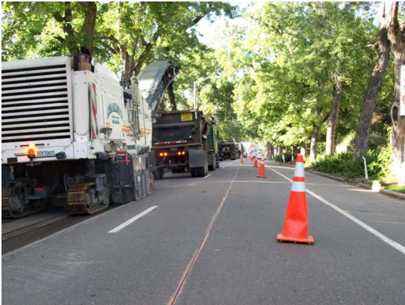
Three inch milling of asphalt between 7 th and 8 th Ave on York St.
