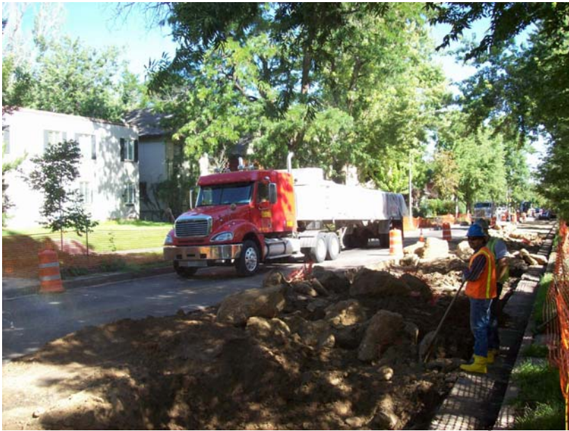
Excavation of utility trenches on York between 12 th and 13 th Ave.
