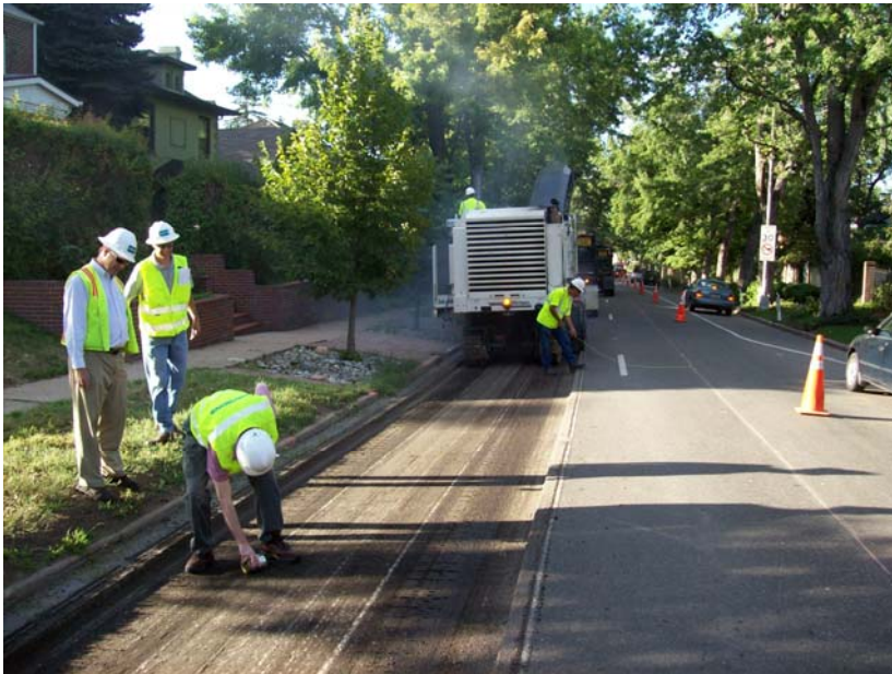
Three inch milling of street between 7 th and 8 th Ave on York St.
