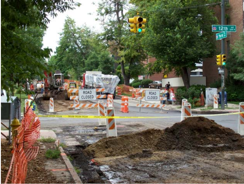
Excavation activities of impacted removal near 12 th and York intersectionl.
