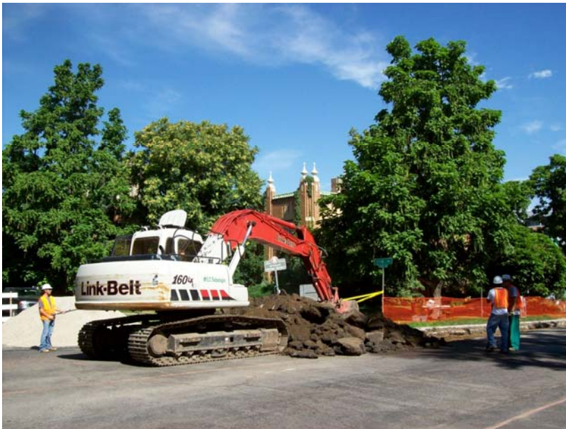
Removal of intersection at 11 th and York St.
