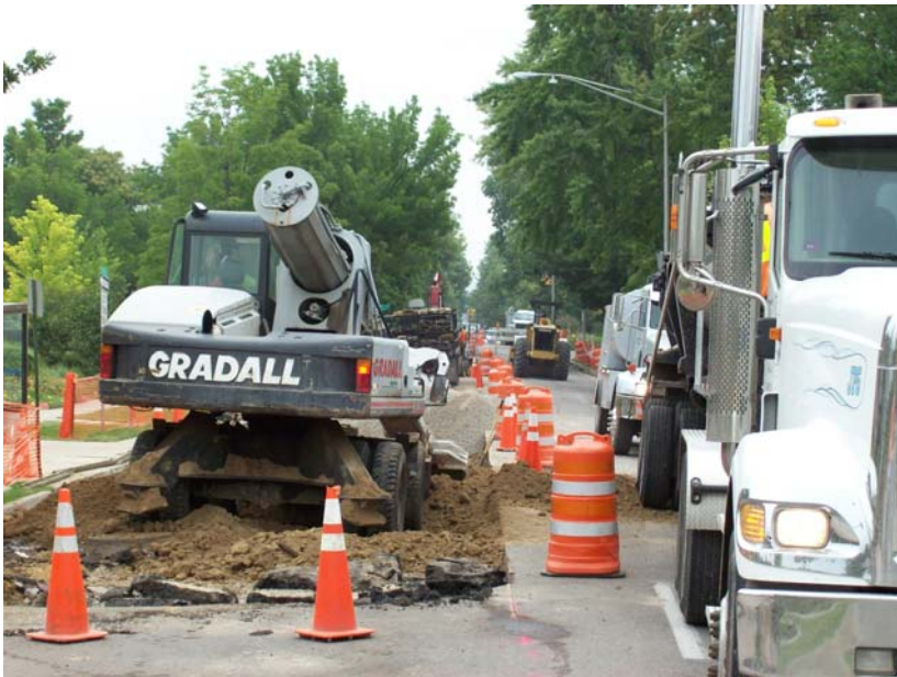
Bus pad reconstruction and grading outside Botanic Gardens on York St.
