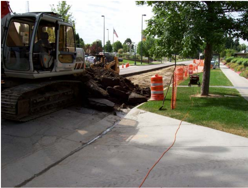
Impacted asphalt removal between 11 th Ave and Botanic Gardens
