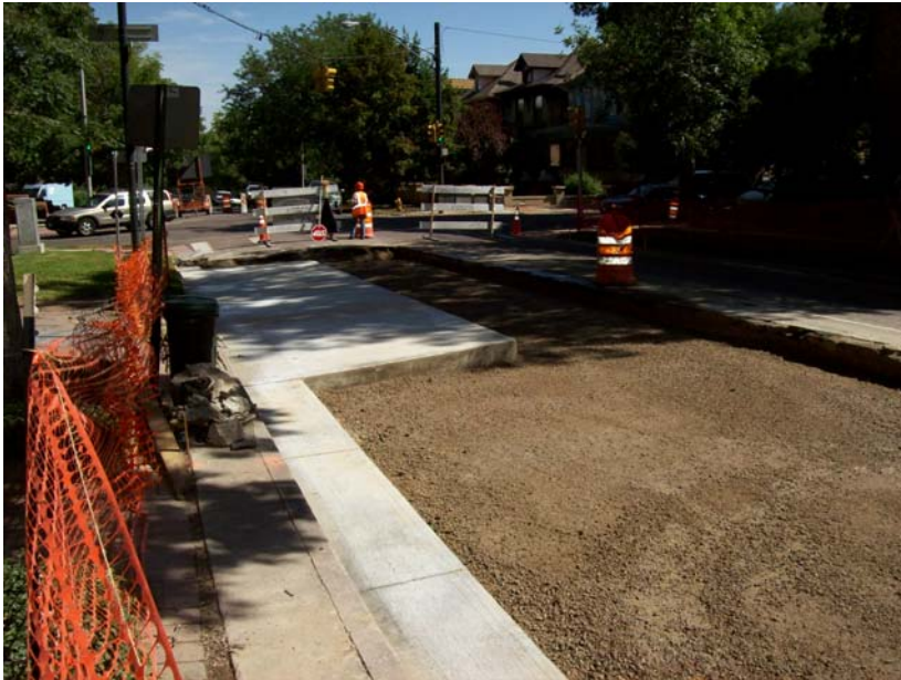
Bus pad reconstruction and grading at 12 th and York St.
