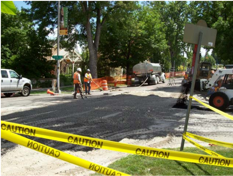
Hot patching of 11 th Ave intersection
