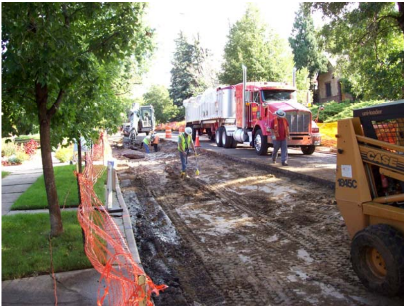
Radiological scanning of subgrade in 600 Block of York St.
