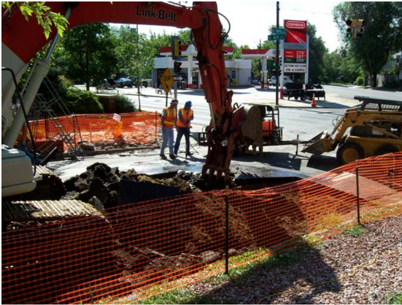
Excavation and removal of impacted asphalt at 6 th Ave intersection.
