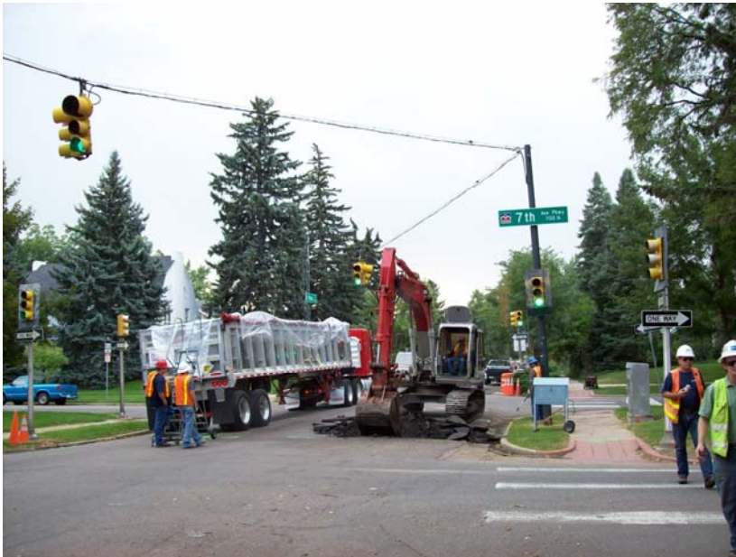
Impacted asphalt removal activities at 7 th Ave and York St.
