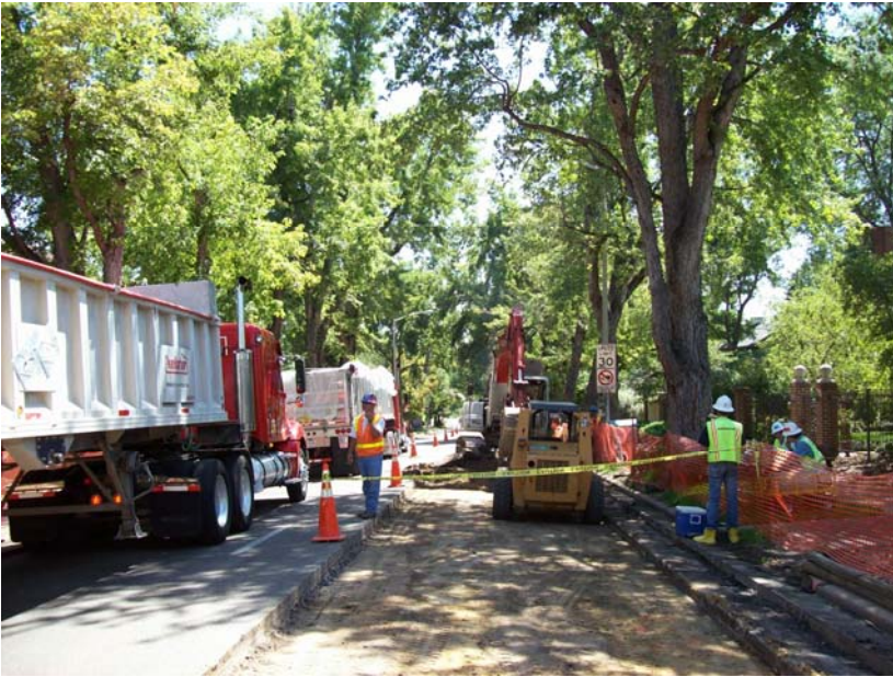
Impacted asphalt removal activities in 800 Block on York St.
