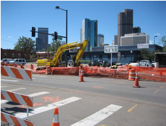
Phase 2 asphalt load out.
