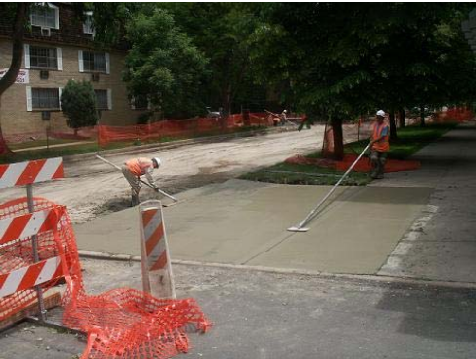
Pouring and finishing new concrete driveway on 9 th Ave.
