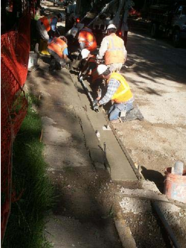
Pouring new curb & gutter on 9 th Ave.
