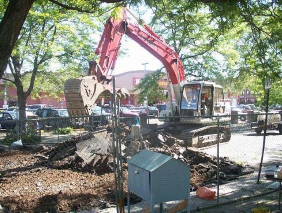
Removing contaminated asphalt on 9 th Ave.
