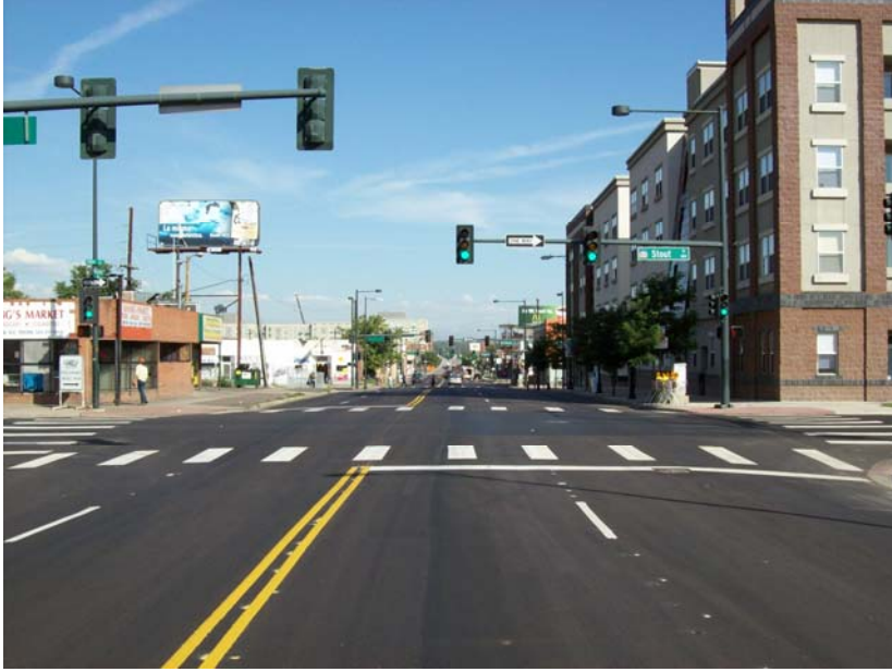
Park Ave at Stout intersection looking west.
