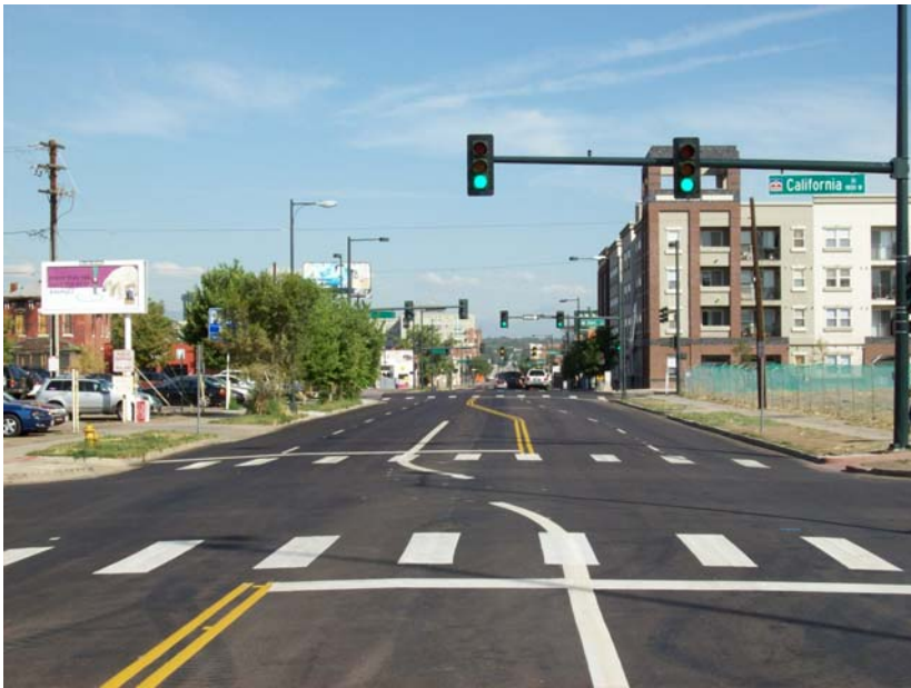
Park Ave at California intersection looking west.
