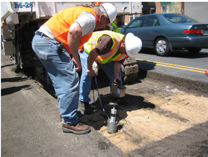
Radium Scanning Activities Along Park Ave.
