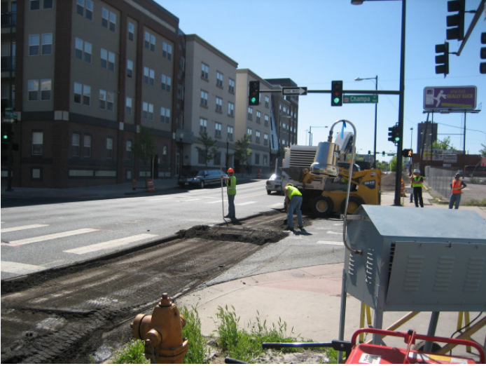
Air monitoring during milling operations.
