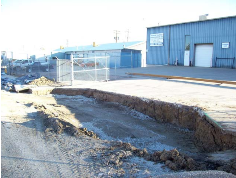
Concrete removal and muck excavation below driveway.
