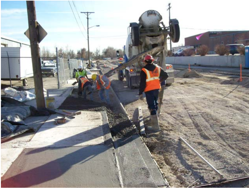
Pouring concrete driveways and curb and gutter.
