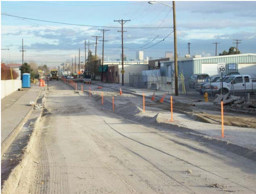
Road reconstruction and grading.
