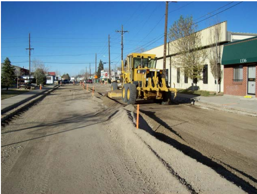
Road reconstruction and grading.
