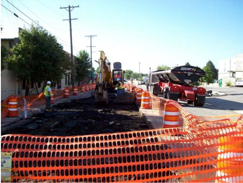
Begin non-impacted asphalt removal in Phase 1.
