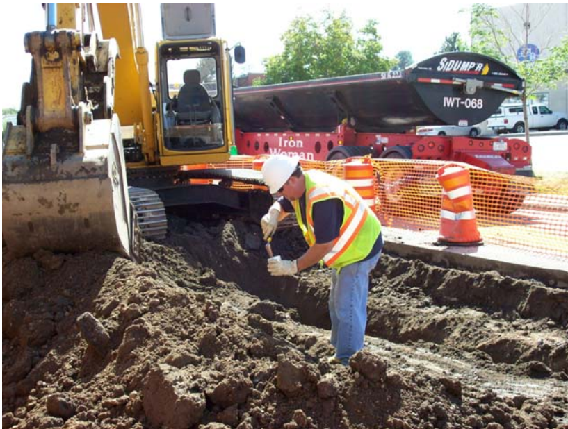
Test Pitting subgrade activities in Phase 1 and 2.
