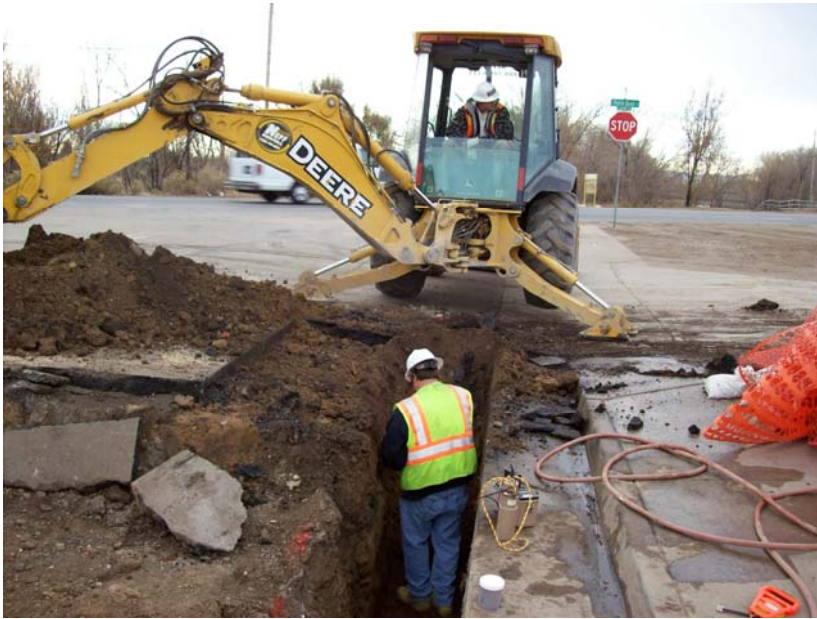
Excavating last of the remaining impacted material in South Jason Street.
