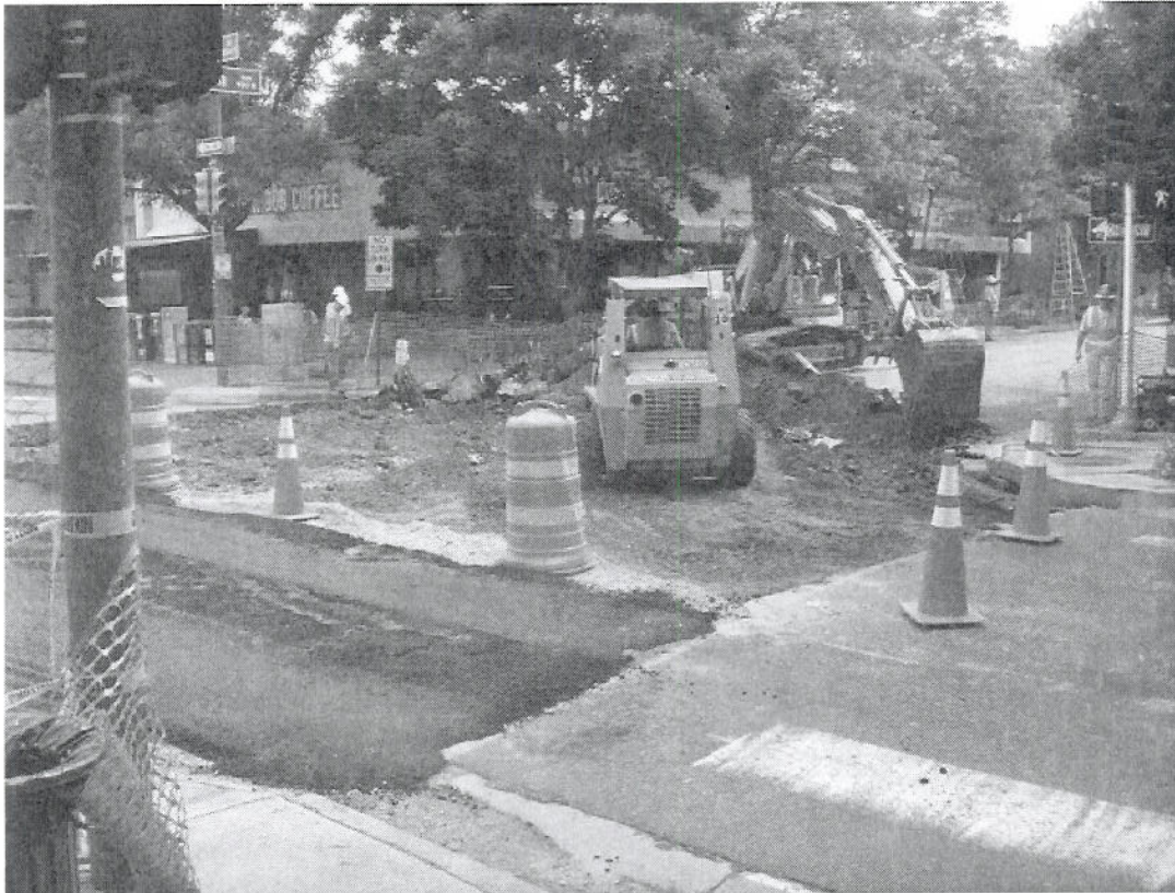
Removal of contaminated asphalt on 9 th Ave.
