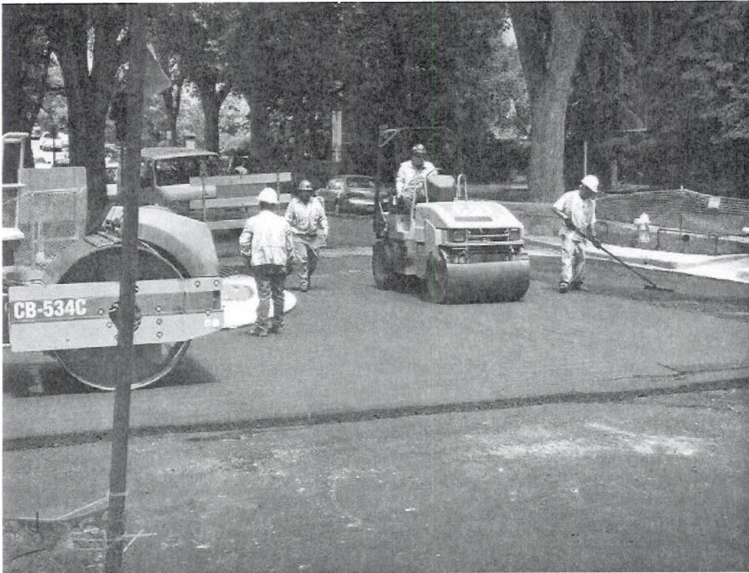
Asphalt paving operations performed on 9 th Ave. & Humboldt St.
