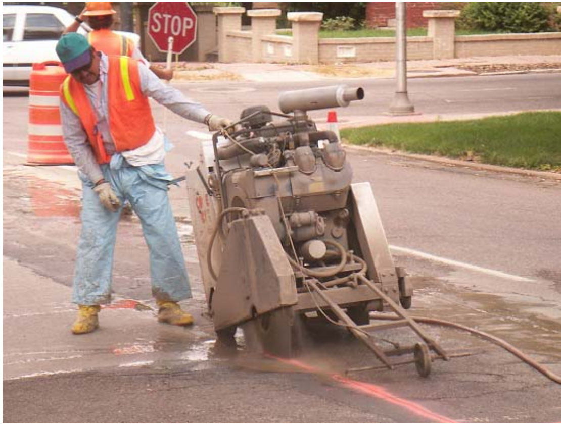
Sawcutting being completed on York Street
