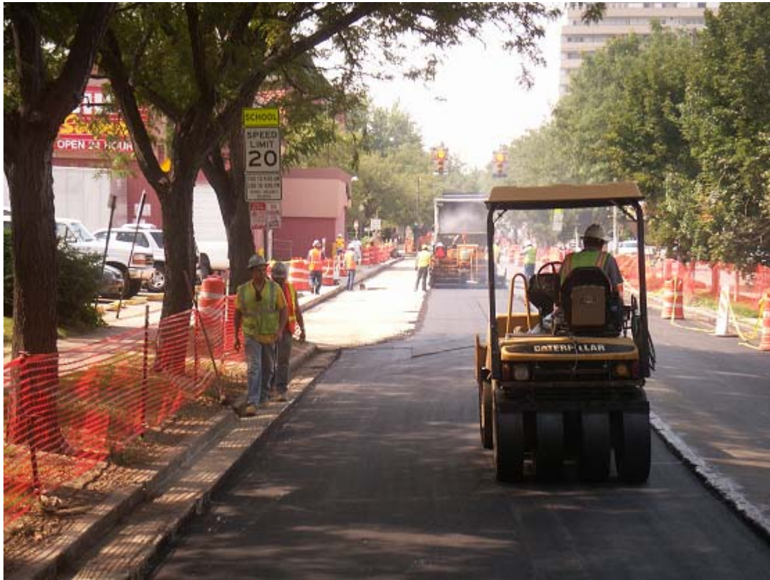
Paving operations being completed on Corona Street
