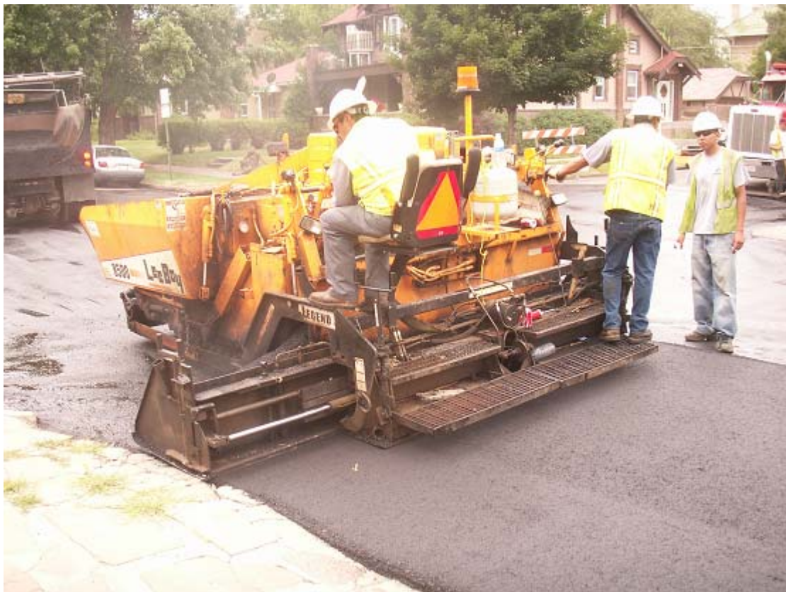
Paving final lift in the intersection of Ogden Street & 9 th Avenue
