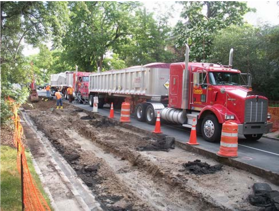
Loading trucks with contaminated asphalt on Corona St.
