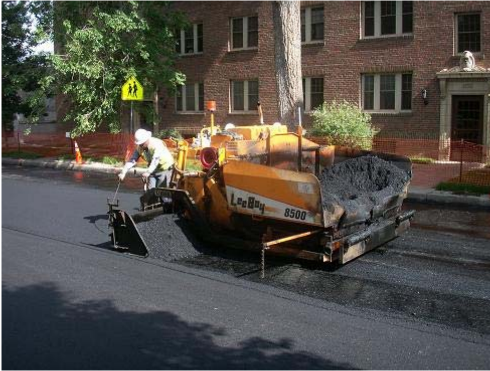
Asphalt paving on 9 th Ave. between Downing St. & Marion St.
