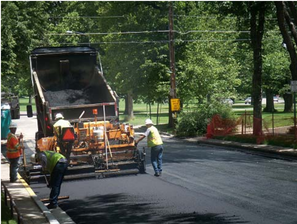
Asphalt paving on 9 th Ave. between Humboldt St. & Cheesman Park
