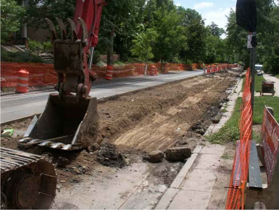
Contaminated asphalt removal on Corona St. between 7 th & 8 th Ave.
