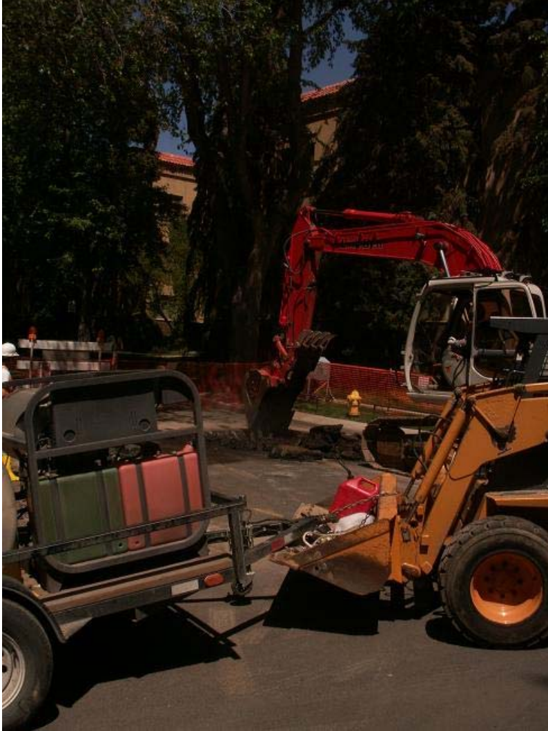
Asphalt removal on 9 th Ave.
