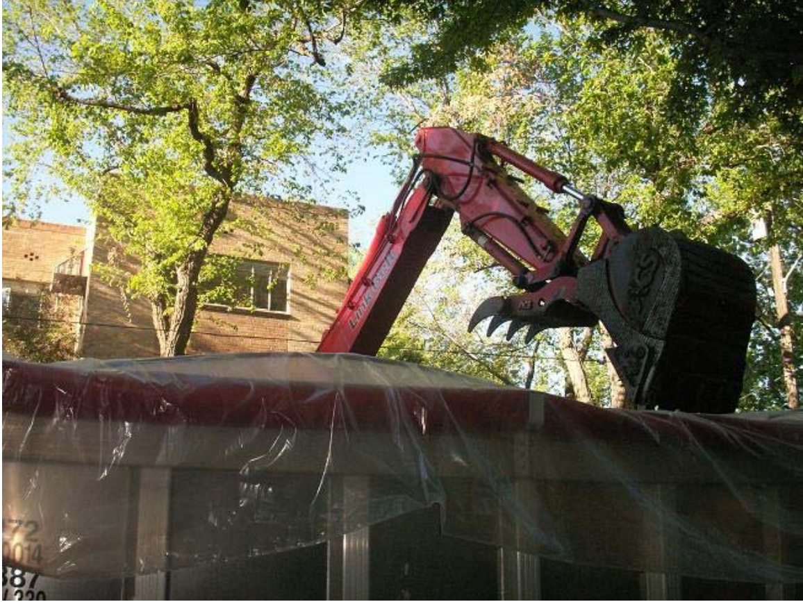
Excavator loading asphalt into lined truck bed
