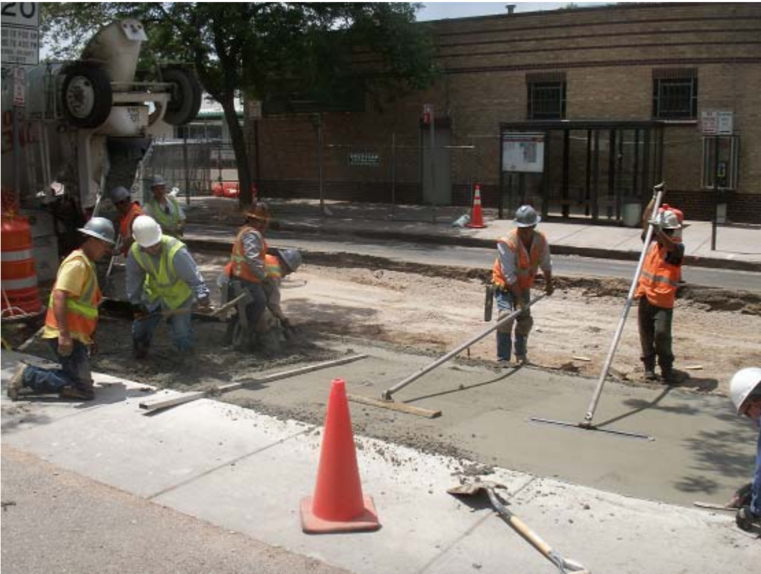
Driveway pan being poured and formed for Moore School on Corona St.
