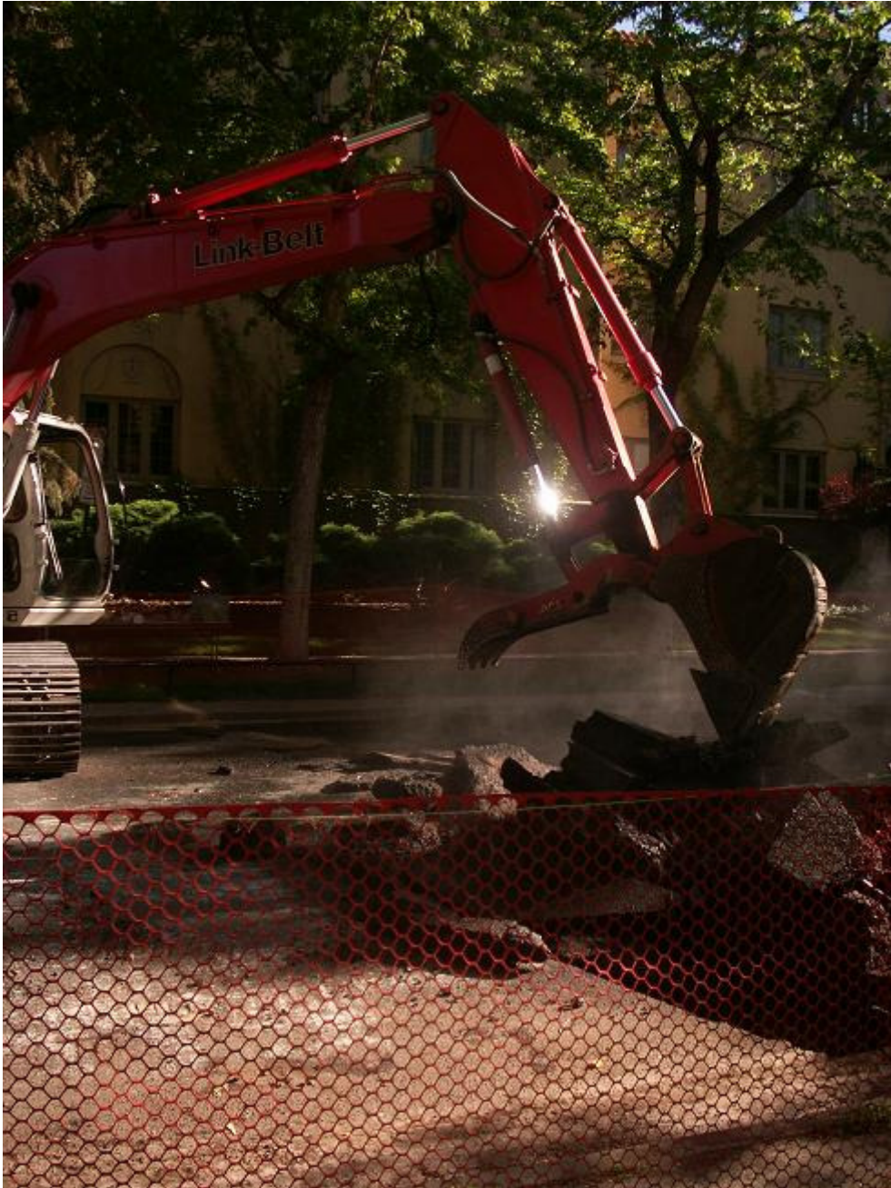
Removing contaminated asphalt from 9 th Avenue
