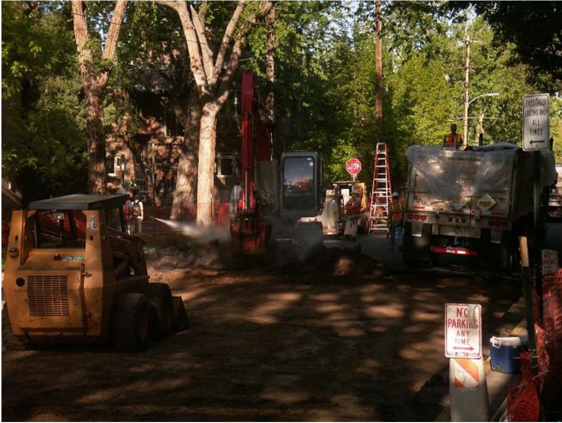
Removing contaminated asphalt from 9 th Avenue
